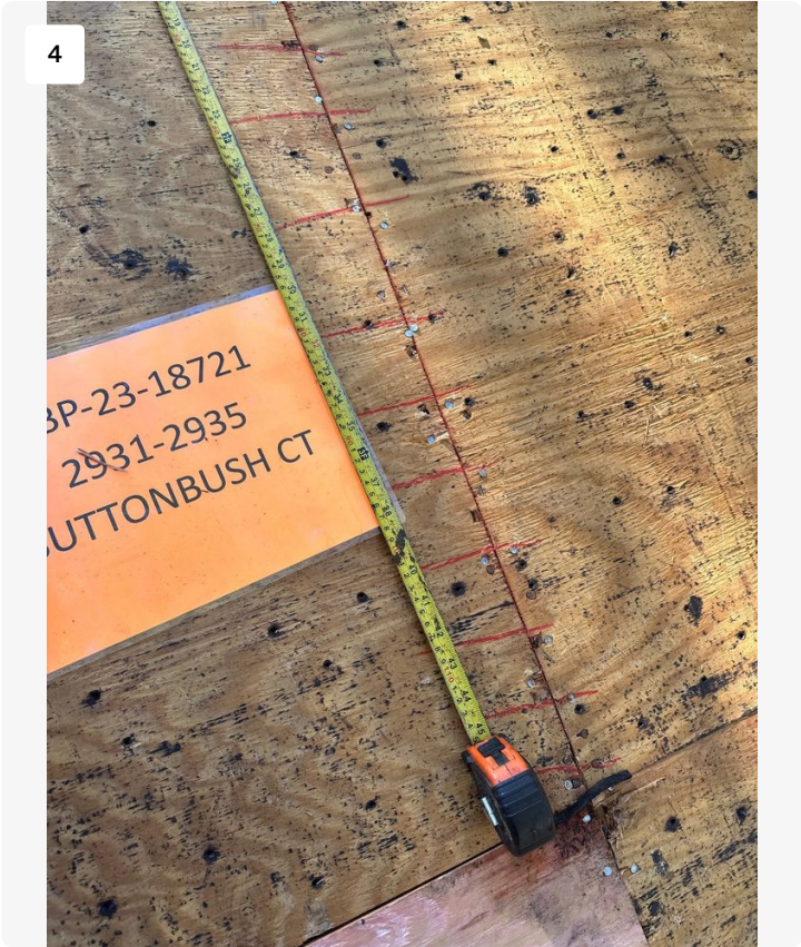
Project: STRATHMORE GATE - 2931-2935 BUTTONBUSH CT / 2310-5005684-01 Date: 2/19/2024, 3:19pm Creator: Maynor Perez
