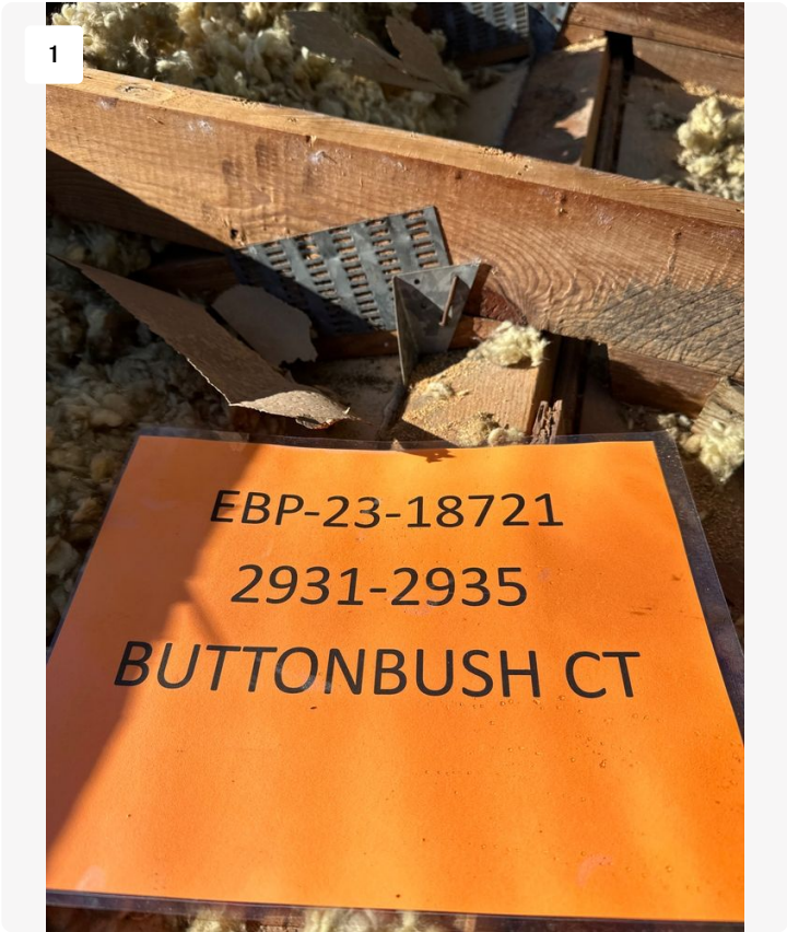
Project: STRATHMORE GATE - 2931-2935 BUTTONBUSH CT / 2310-5005684-01 Date: 2/19/2024, 3:01pm Creator: Maynor Perez
