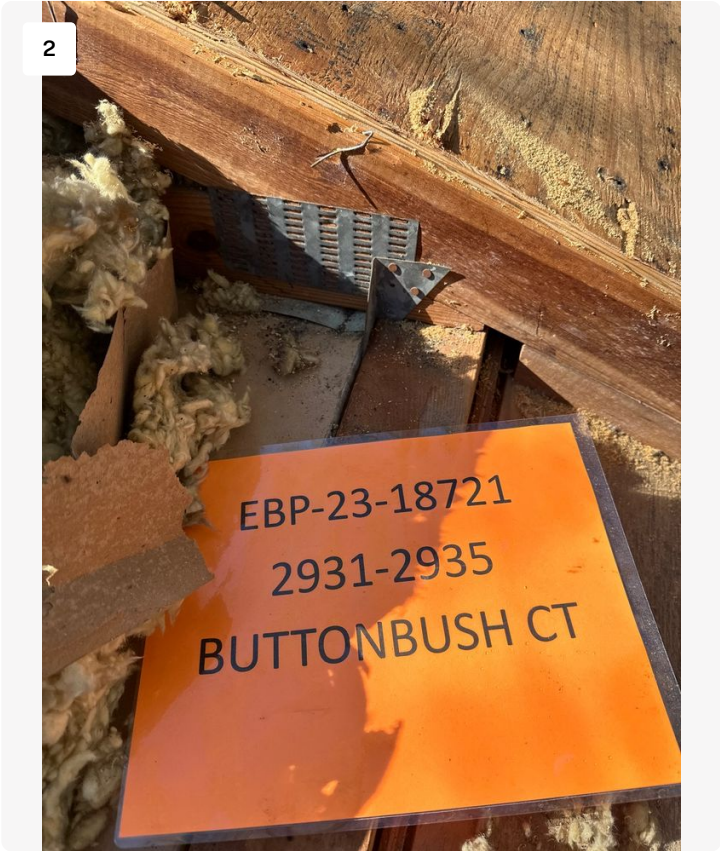
Project: STRATHMORE GATE - 2931-2935 BUTTONBUSH CT / 2310-5005684-01 Date: 2/19/2024, 3:02pm Creator: Maynor Perez
