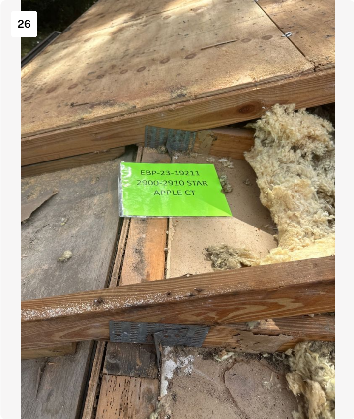
Project: STRATHMORE GATE -2900-2910 STAR APPLE CT / 2310-5006484-01 Date: 12/11/2023, 11:52am Creator: Maynor Perez
