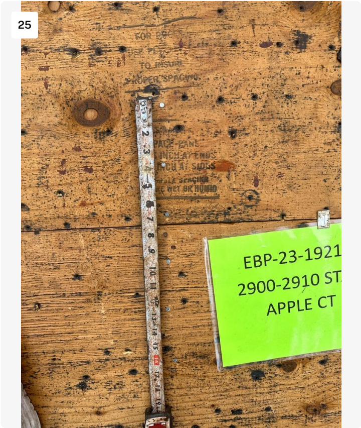
Project: STRATHMORE GATE -2900-2910 STAR APPLE CT / 2310-5006484-01 Date: 12/12/2023, 11:32am Creator: Maynor Perez
