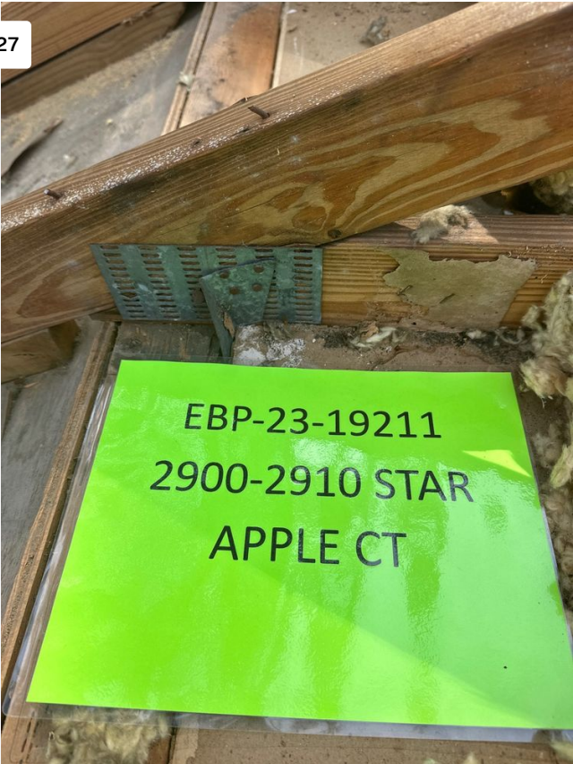
Project: STRATHMORE GATE -2900-2910 STAR APPLE CT / 2310-5006484-01 Date: 12/11/2023, 11:51am Creator: Maynor Perez
