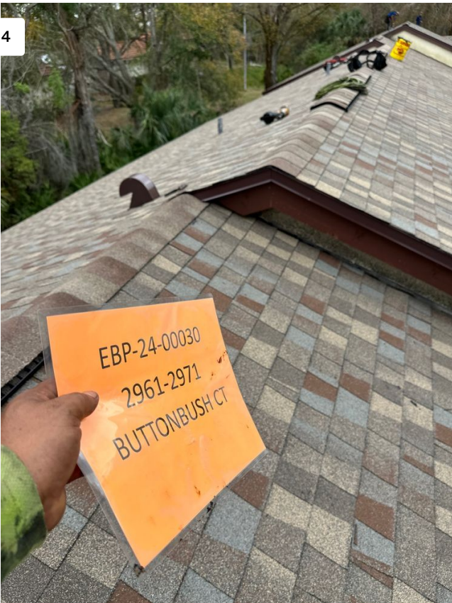
Project: STRATHMORE GATE - 2961-2971 BUTTONBUSH CT / 2310-5006192-01 Date: 2/15/2024, 1:35pm Creator: Maynor Perez
