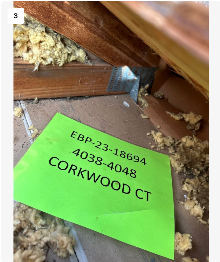
Project: STRATHMORE GATE - 4038-4048 CORKWOOD CT / 2310-5005592-01 Date: 1/23/2024, 9:25am Creator: Maynor Perez
