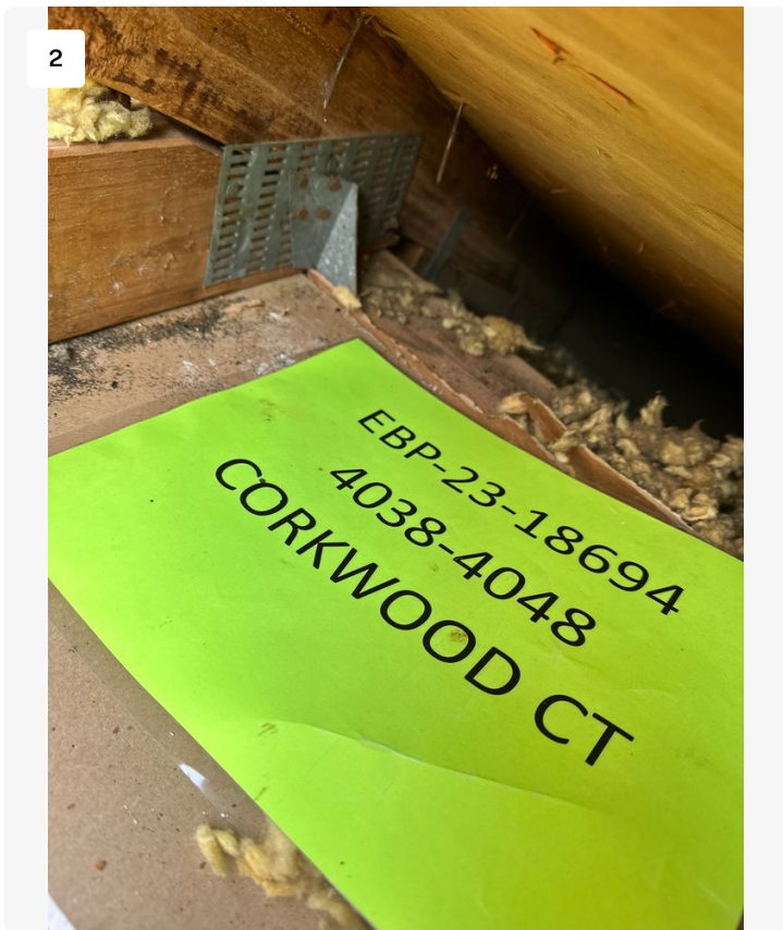
Project: STRATHMORE GATE - 4038-4048 CORKWOOD CT / 2310-5005592-01 Date: 1/23/2024, 9:24am Creator: Maynor Perez
