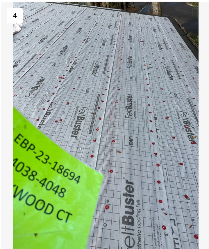
Project: STRATHMORE GATE - 4038-4048 CORKWOOD CT / 2310-5005592-01 Date: 1/24/2024, 9:16am Creator: Maynor Perez
