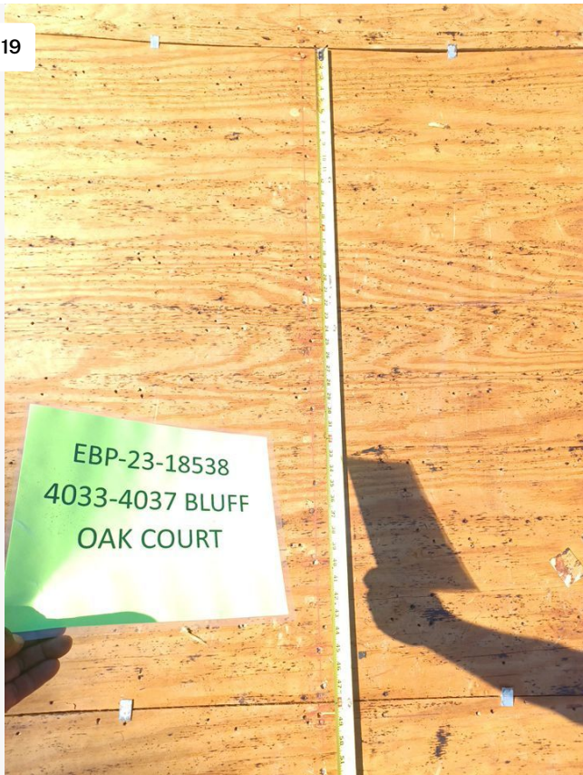
Project: STRATHMORE GATE - 4033-4037 BLUFF OAK CT / 2310-5005455-01 Date: 11/20/2023, 12:06pm Creator: Lucio Roofer
