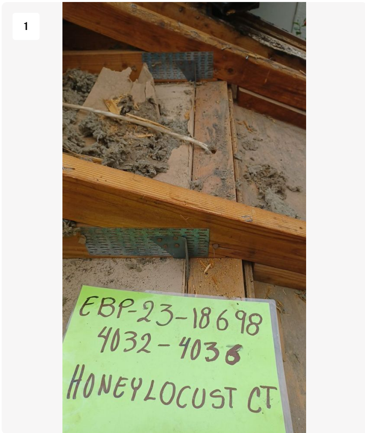
Project: STRATHMORE GATE - 4032-4036 HONEYLOCUST CT / 2310-5005622-01 Date: 1/8/2024, 10:50am Creator: Lucio Roofer
