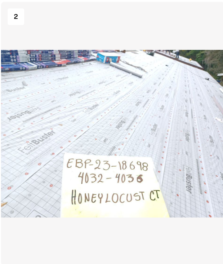
Project: STRATHMORE GATE - 4032-4036 HONEYLOCUST CT / 2310-5005622-01 Date: 1/8/2024, 11:36am Creator: Lucio Roofer
