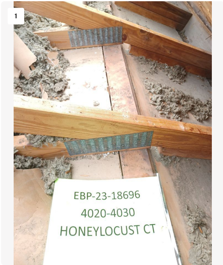
Project: STRATHMORE GATE - 4020-4030 HONEYLOCUST CT / 2310-5005605-01 Date: 1/16/2024, 9:31am Creator: Lucio Roofer
