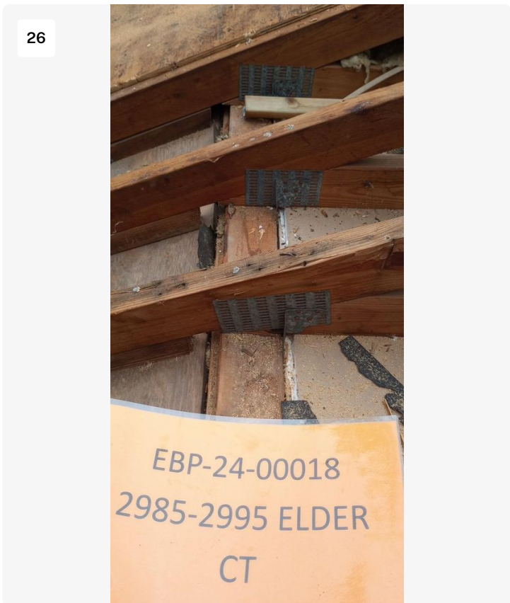
Project: STRATHMORE GATE -2985-2995 ELDER CT / 2310-5007237-01 Date: 1/30/2024, 5:24pm Creator: Lucio Roofer
