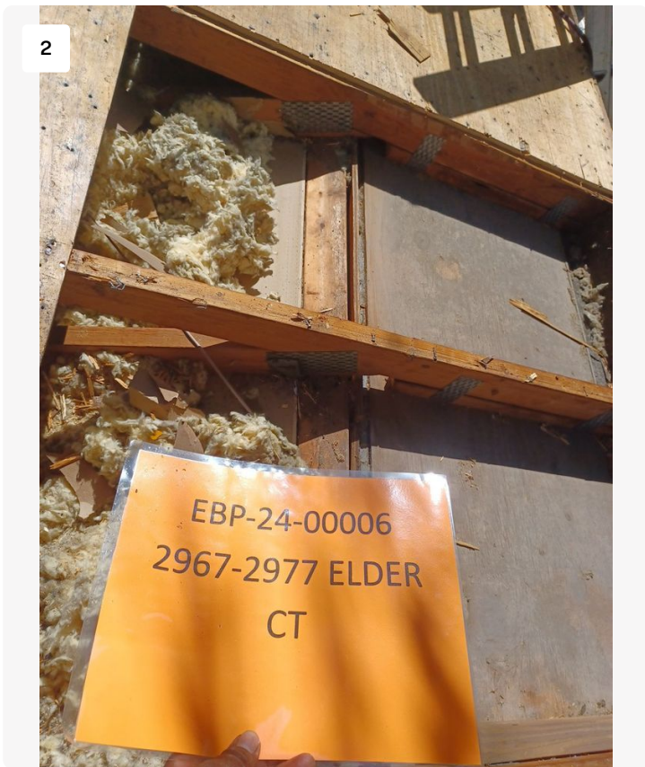
Project: STRATHMORE GATE -2967-2977 ELDER CT / 2310-5006567-01 Date: 2/6/2024, 1:46pm Creator: Lucio Roofer
