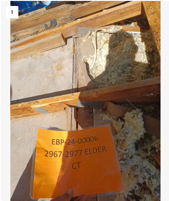
Project: STRATHMORE GATE -2967-2977 ELDER CT / 2310-5006567-01 Date: 2/6/2024, 1:45pm Creator: Lucio Roofer
