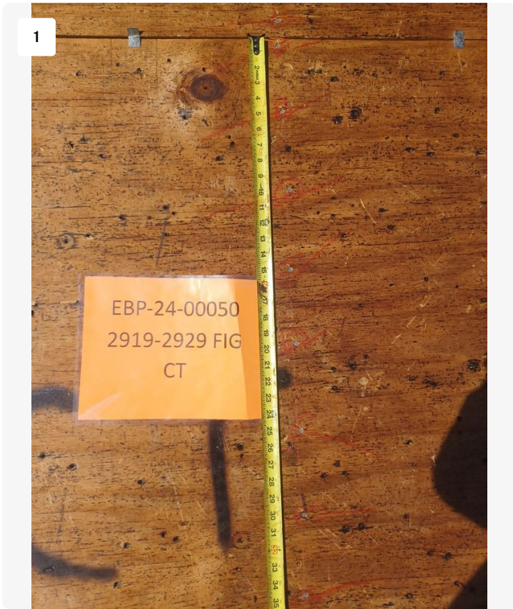
Project: STRATHMORE GATE -2919-2929 FIG CT / 2310-5006264-01 Date: 2/26/2024, 2:21pm Creator: Lucio Roofer
