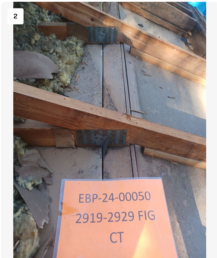
Project: STRATHMORE GATE -2919-2929 FIG CT / 2310-5006264-01 Date: 2/26/2024, 4:07pm Creator: Lucio Roofer
