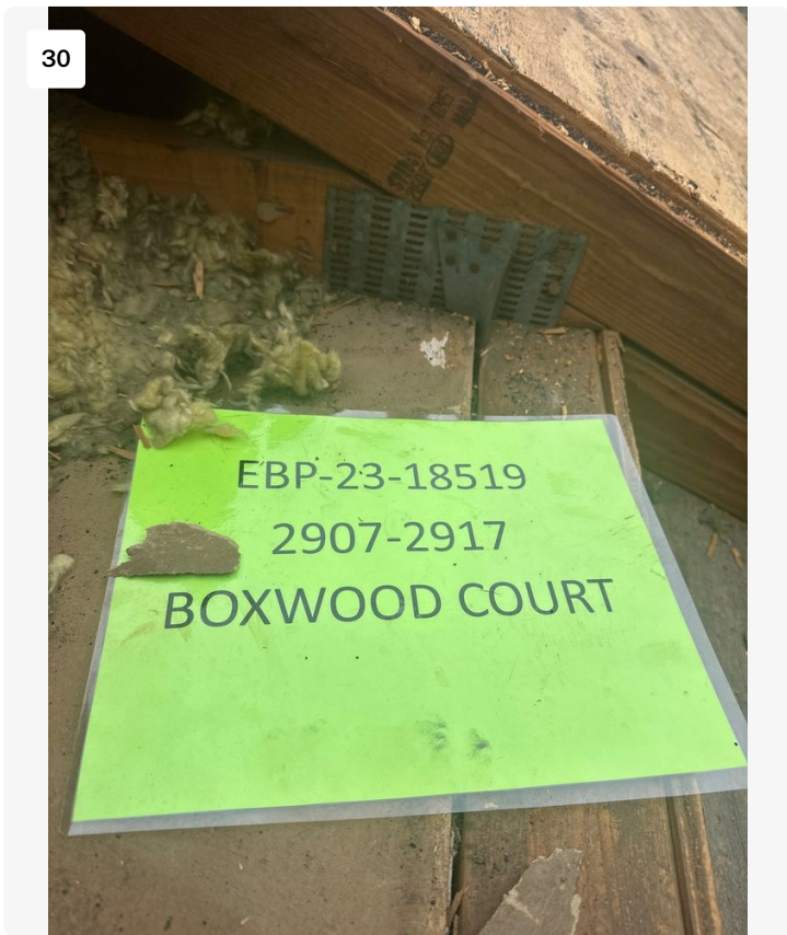
Project: STRATHMORE GATE -2907-2917 BOXWOOD CT / 2310-5007341-01 Date: 11/28/2023, 1:41pm Creator: Maynor Perez
