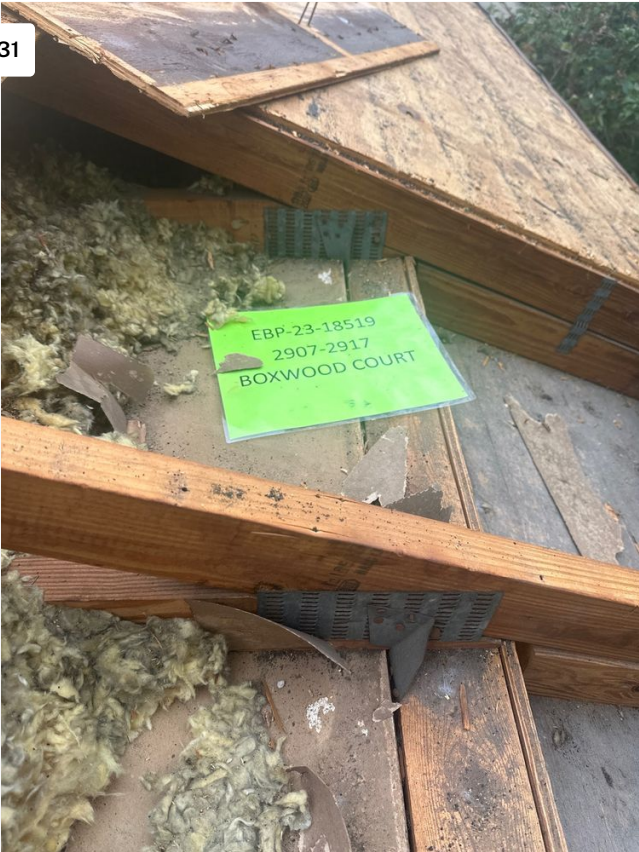
Project: STRATHMORE GATE-2907-2917 BOXWOOD CT / 2310-5007341-01 Date: 11/28/2023, 1:41pm Creator: Maynor Perez
