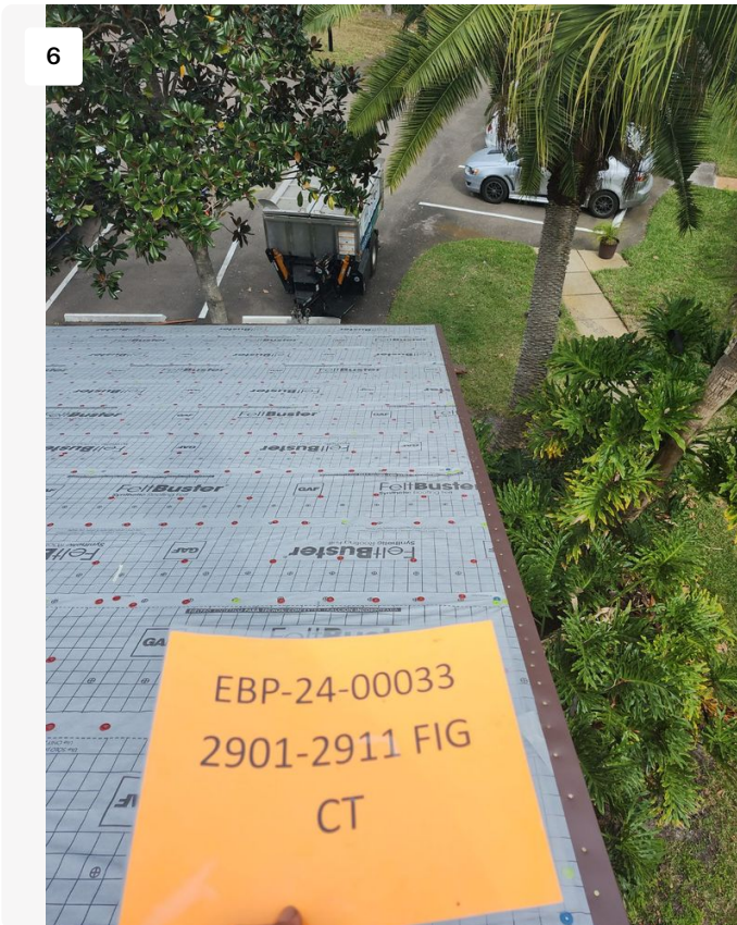
Project: STRATHMORE GATE - 2901-2911 FIG CT / 2310-5006206-01 Date: 3/5/2024, 11:53am Creator: Lucio Roofer
