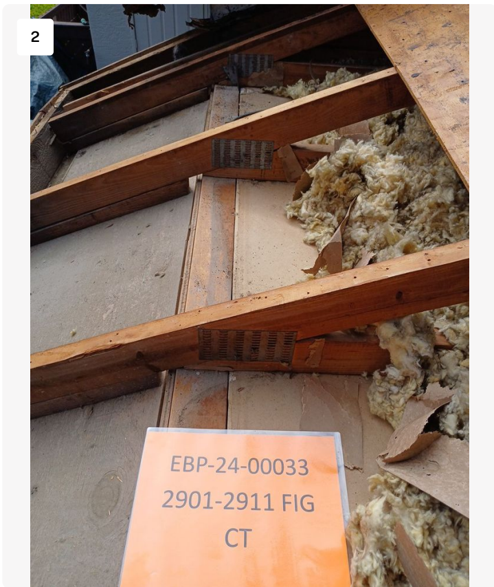
Project: STRATHMORE GATE -2901-2911 FIG CT / 2310-5006206-01 Date: 3/4/2024, 9:59am Creator: Lucio Roofer
