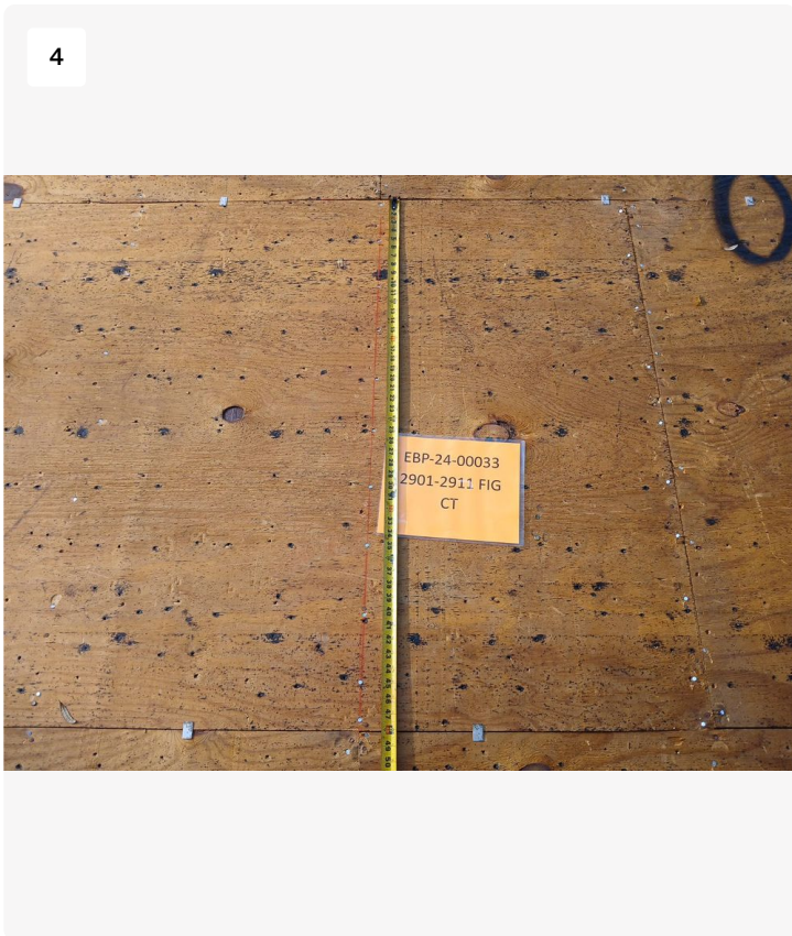
Project: STRATHMORE GATE - 2901-2911 FIG CT / 2310-5006206-01 Date: 3/4/2024, 4:31pm Creator: Lucio Roofer
