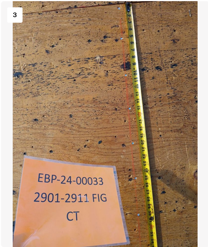
Project: STRATHMORE GATE - 2901-2911 FIG CT / 2310-5006206-01 Date: 3/4/2024, 4:30pm Creator: Lucio Roofer
