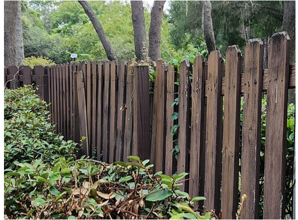
Damaged wood fence at pool area
